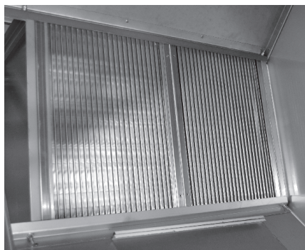
Plate recuperator (Fig. 12)
